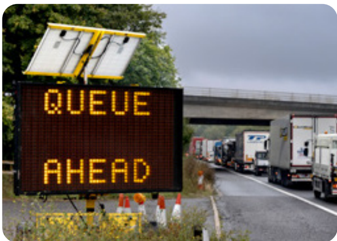
▲ VMS triggered to warn drivers of queuing traffic
